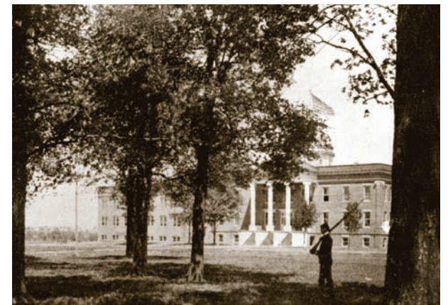
The MMA campus circa 1901 consisted of the main administration building and two residence halls.
